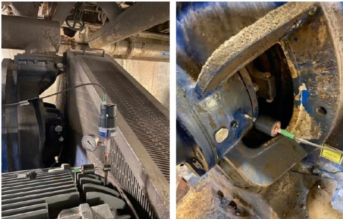
Figure 1 & 2: DE & NDE ConMonSense Sensor & Grease Cartridge Configuration
